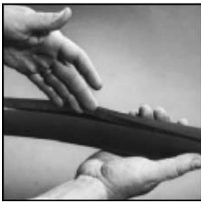
FIG. 3 Apply Unslit Insulation to Straight Pipe
