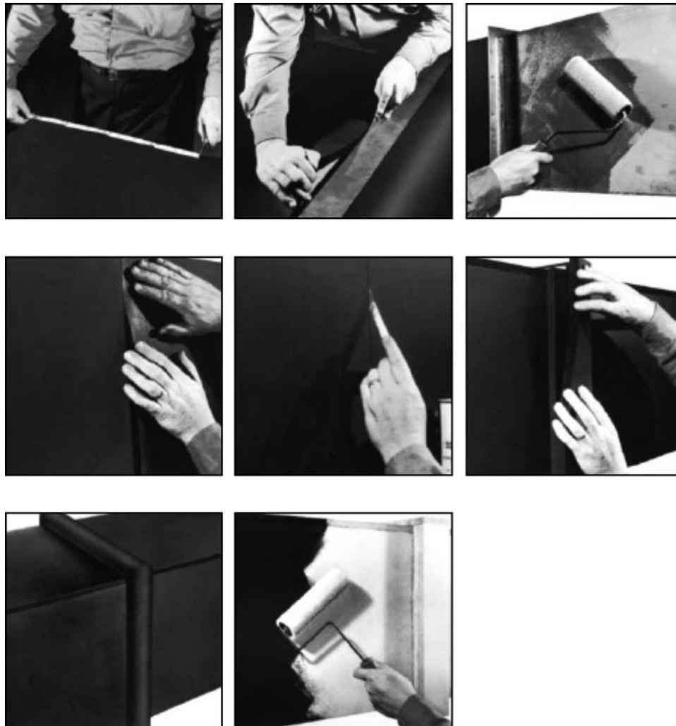
FIG. 13 Duct Covering
